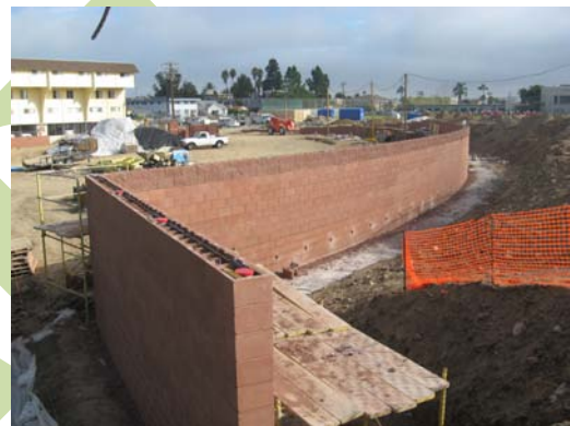
New retaining wall for Girl's Softball Field at Hoover HS
