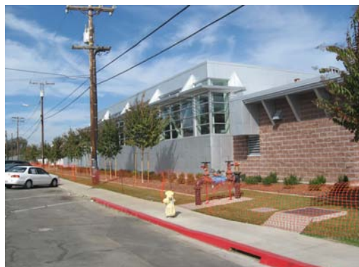
Hoover HS: New construction includes a landscaped perimeter
